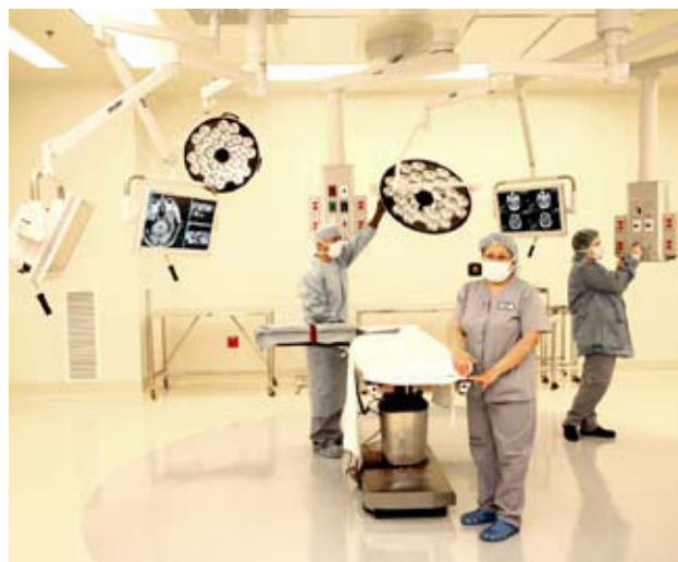
One of two new state-of-the-art OR suites at Northridge Hospital
